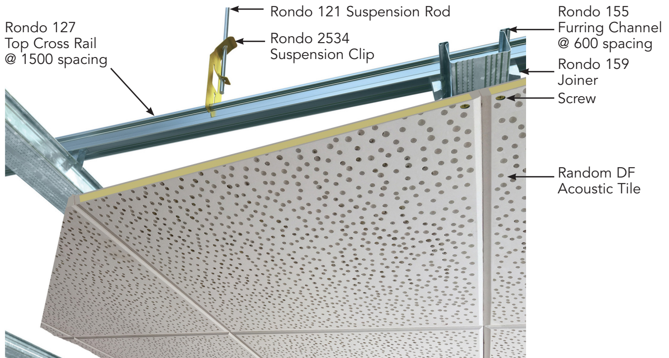
BOTTOM VIEW Typical Ceiling Installation with RONDO KEY-LOCK® Ceiling System
