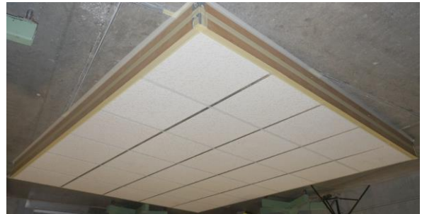
Test specimen installed for testing (image inverted to depict ceiling installation)
